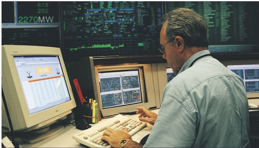
[4] A coordinator [above] in the control room of the California Independent System Operator monitors status of generators, lines, and loads. Before the establishment of the ISO, there was no one central control room providing a complete overview of the state's grid. The control room's head, Ed Riley [right], believes the new setup will go far to prevent the kinds of outages that occurred in 1996 in the Western Interconnection.
